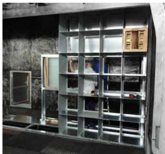
Step2 - retrofitting: Slide-in elements are assembled to bear edrizzi® paint mist separators and secondary filters NFEWP03.
