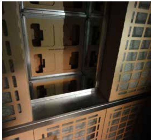
Step4 - retrofitting: Rear view of separation wall fully equipped with edrizzi® VARIO and NFEWP03.
