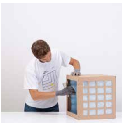
Step 3: The filter medium is fixed with a tackers, the straps at the top are latched for stability and the box is closed. The completely ready box is pushed into the holding frame.
