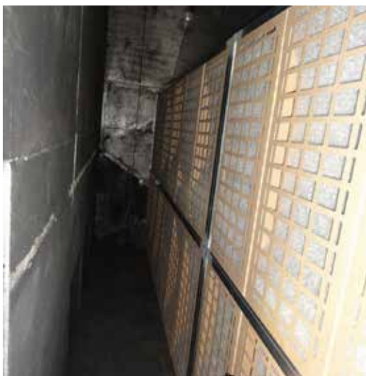
Step5 - retrofitting completed: The depression chamber.
