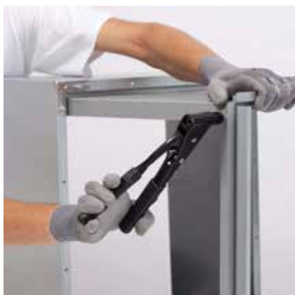
Step 6: The last bracket is fixed with rivets only at this stage.
