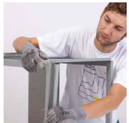
Step 5: Attention: Before the last bracket is fixed with rivets, hook the locking bar behind at the top and bottom of the holes provided for this purpose.
