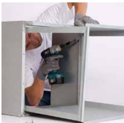
Step 4: The cover is fixed with self-tapping screws to the slide-in element.
