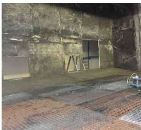
Step1 - retrofitting: Waterwall is removed, depression chamber lays bare.
