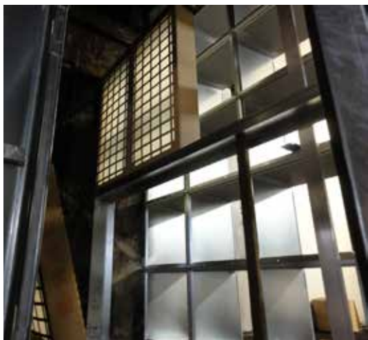
Step3 - retrofitting: Rear view of edrizzi® wall including paint mist separators and secondary filter elements NFEWP03.
