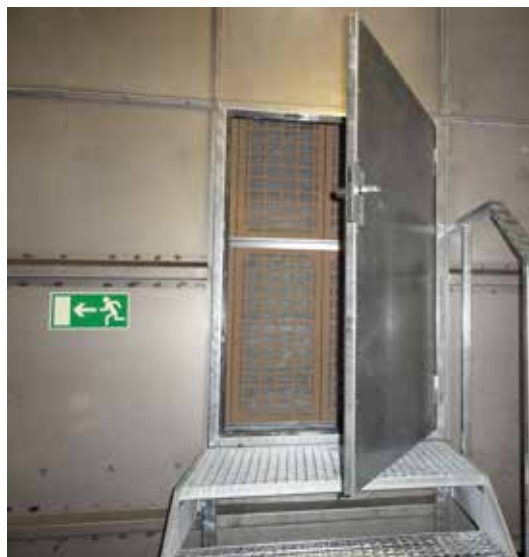
Step6 - retrofitting completed: Rear door to depression chamber for secondary filter change.
