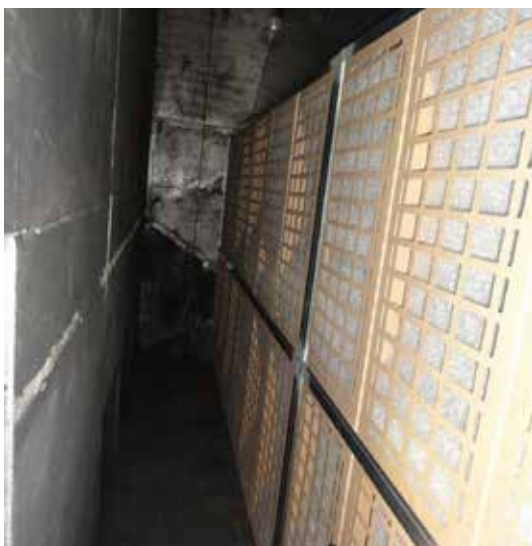
Step5 - retrofitting completed: The depression chamber.
