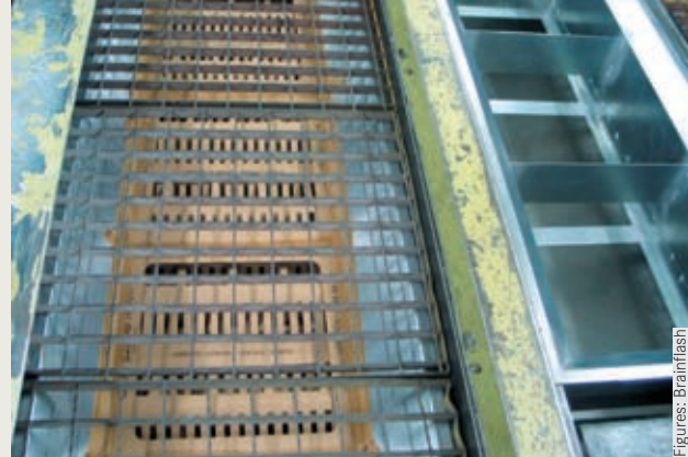
The dry filter system is installed in pre-manufactured steel frame support structures that are hung into place before a conversion is carried out
